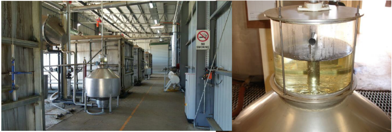
Figure 5: Tea tree distillery (L) and tea tree oil in a separator apparatus post-distillation (R)
